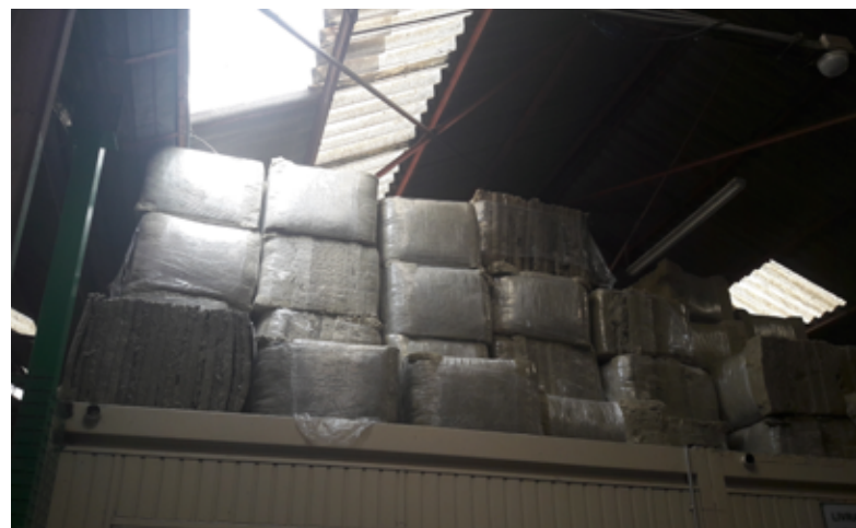
Storage of mineral wool insulation from interior partitions, before reuse as sloping roof insulation
