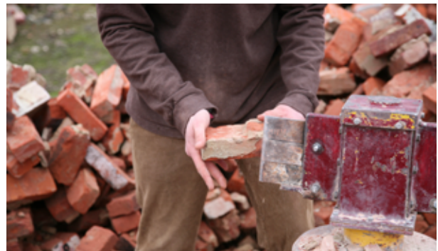
Manual and mechanical cleaning of mortar remains
