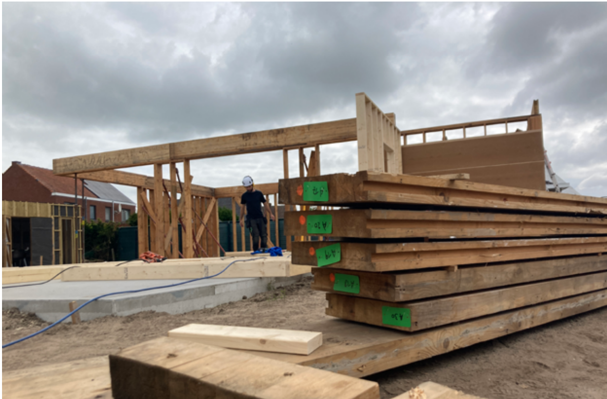
Example of marks applied to beams of laminated wood © HuisMus - Trovo
