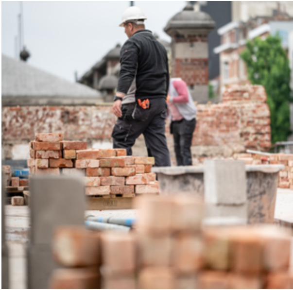
Removing bricks – Ixelles barracks
