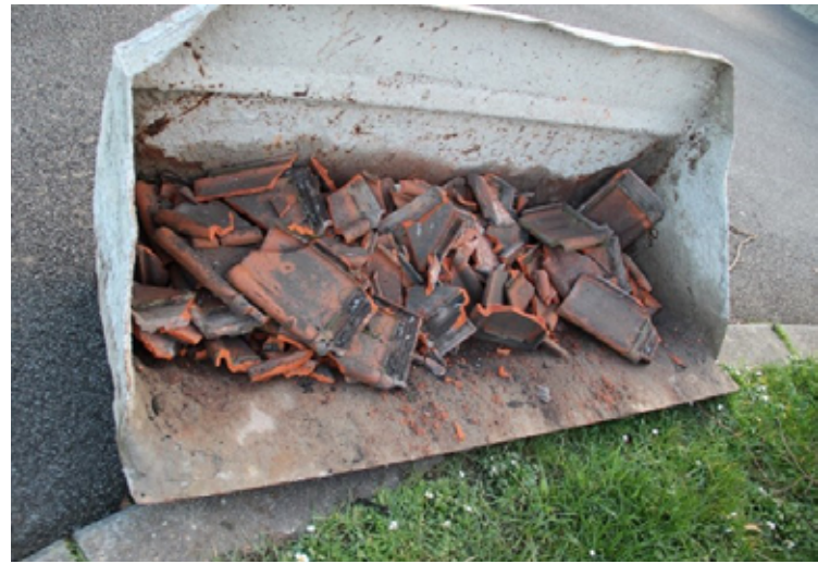
Example of sorting of remains of tiles not reusable during removal
